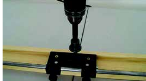
Fig.7. Drilling lead hole with d.12,5 drill.
