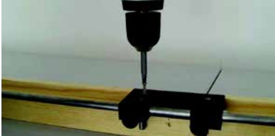
Fig.6. Screwing down frame with screws.
